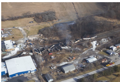
An aerial view of the NS train derailment in East Palestine, Ohio taken on February 5, 2023. 5
