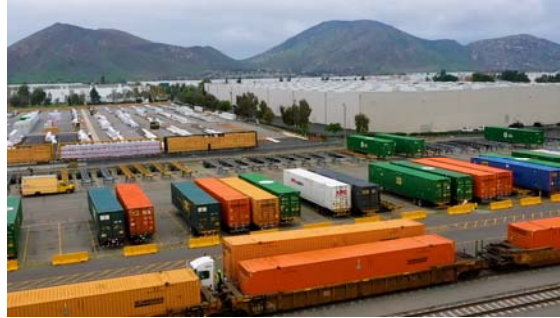
Inland Empire Intermodal Terminal Colton, California
